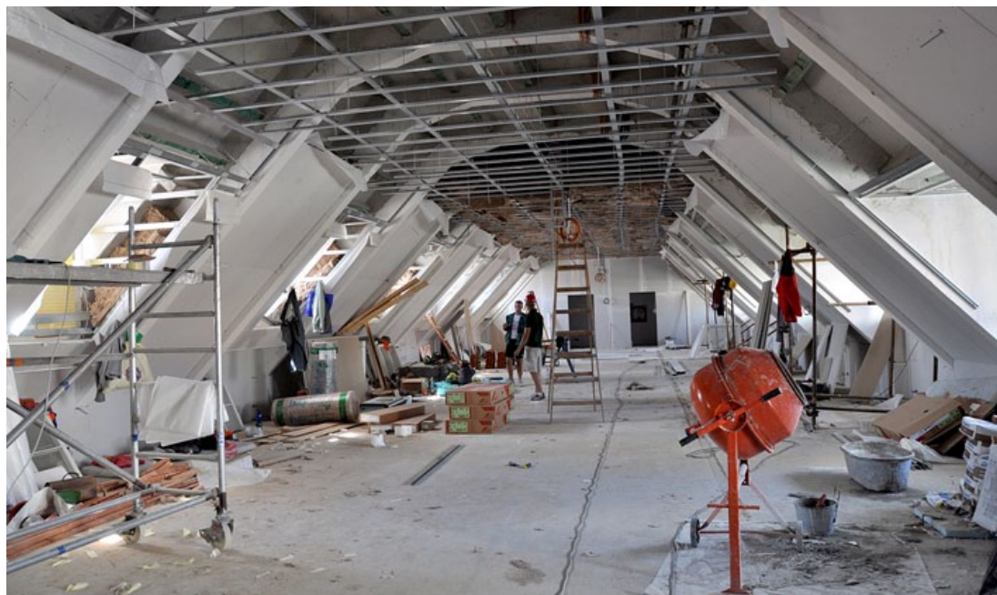
Insulation of the attic depository. Photo: Pavel Macenauer
